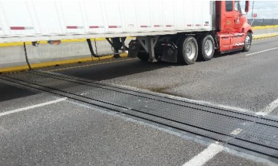
ISOSISM® SFX under heavy traffic loads – Puebla Viaduct (Mexico)
