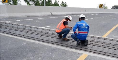
ISOSISM® SFX inspection on Sentul Selatan viaduct (Indonesia)
